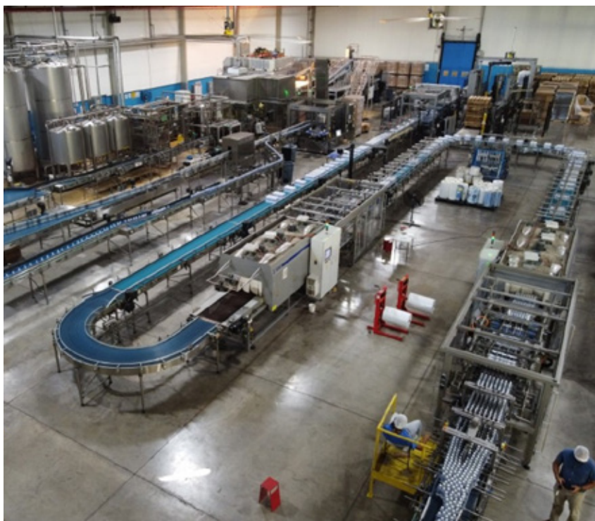
'Wata' plant at Wisynco's Lakes Pen location.
